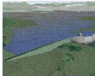
Aerial view of the new Spring Grove Dam that is currently under construction
